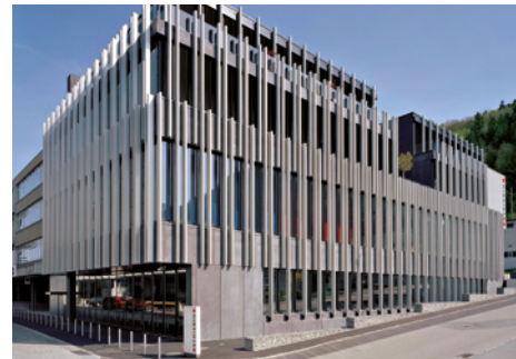
Vertically structured - the facade of the corporate headquarters in Littau near Lucerne
